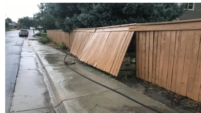
The culvert crossing of Westerly Spring Creek at East Phillips Avenue clogged, resulting in flows overtopping the road damaging private property and an electric transformer in the area
