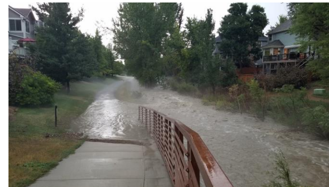
Pedestrian trails were inundated along Spring Creek downstream of East Mineral Avenue
