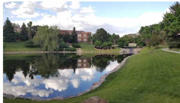
Yosemite Pond provides stormwater detention as well as a water feature
