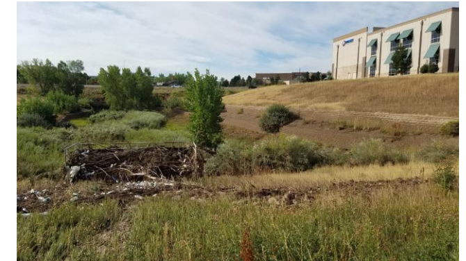
Significant debris collected at Spring Creek Detention Basin but the facility did not overtop County Line Road
