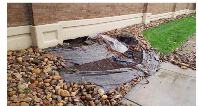
Localized flooding caused damage to landscaping rock on South Holly Street near East Kettle Avenue
